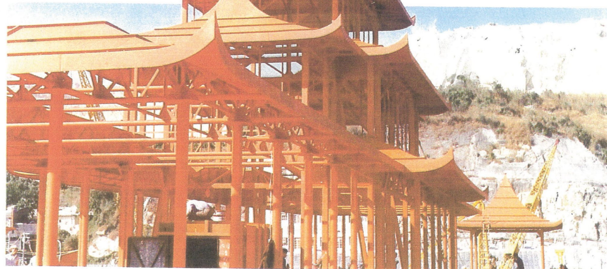
Construction of Jumbo Floating Restaurant, 1976
